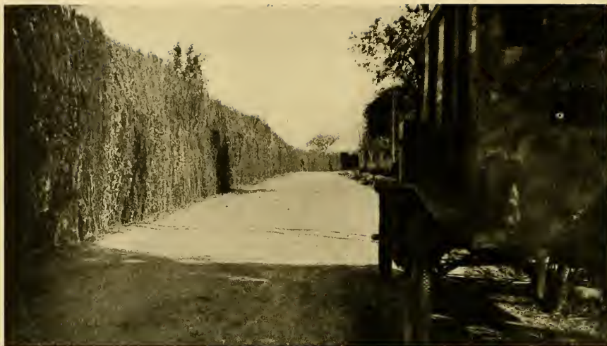
A camouflaged road near Pont à Mousson
